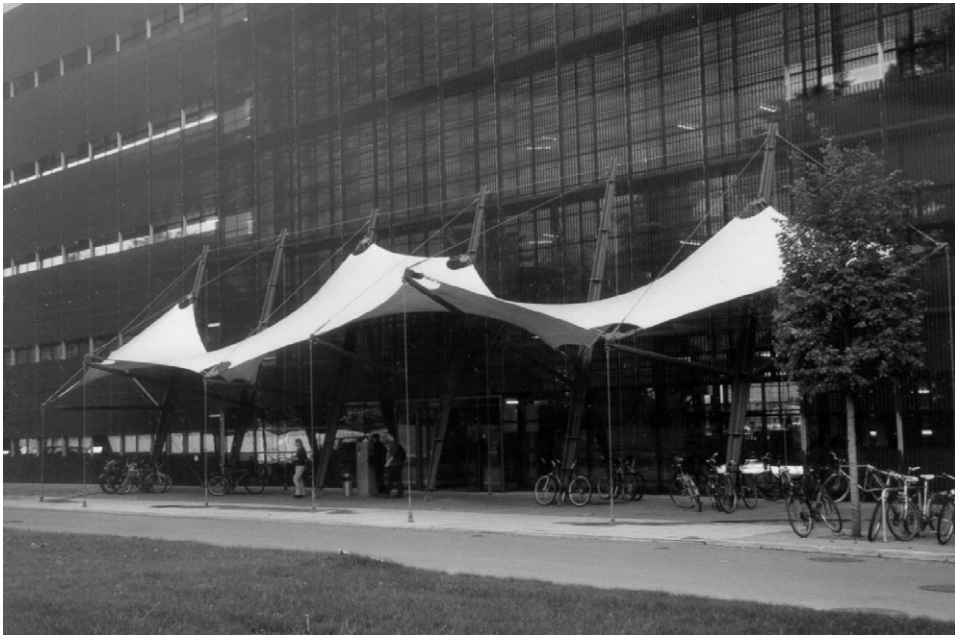
Fig. 32. Geometry of the membranous roof.
